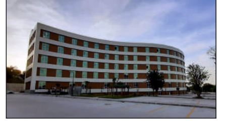
Etimesgut 250 Yataklı Devlet Hastanesi Etimesgut 250-Bed State Hospital
