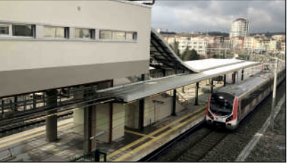
Marmaray GYH Metro Marmaray GYH Subway Line
