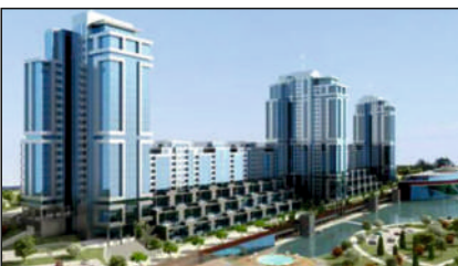
Akfen İncek Loft Akfen İncek Loft Residential Buildings
