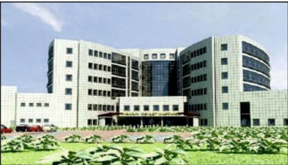
Aksaray 400 Yataklı Devlet Hastanesi Aksaray 400-Bed State Hospital
